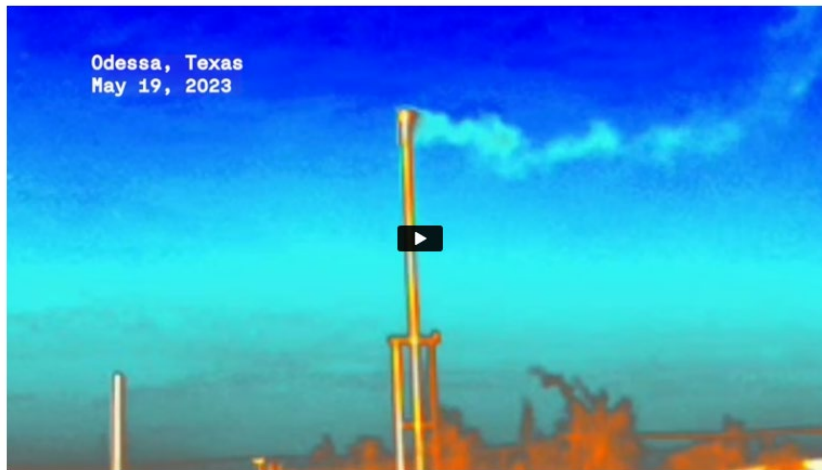
An unlit flare leaks gas, as shown in an infrared video taken by state inspectors on May 19, 2023, across the street from the Hinojos family home in Odessa, Texas. Footage obtained by public records request.
