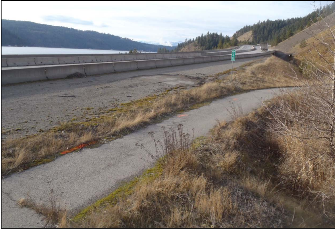
Photo 5. Looking northwest at I-90 and top of existing 8-foot asphalt pathway. Connection to the highway would be at mile marker 20 (green sign). During transports, the concrete Jersey barriers along the near side and median of the highway would be temporarily removed. The Jersey barriers would not be removed during on-ramp construction.
