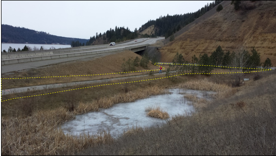
Photo 1. Looking southwest at existing 8-foot wide asphalt pathway and ITD Drainage Pond. Proposed temporary on-ramp will be centered on the pathway. The ITD Drainage Pond will not be disturbed and will be protected during construction with erosion and sediment control measures. On-ramp footprint would be within yellow dashed line.
