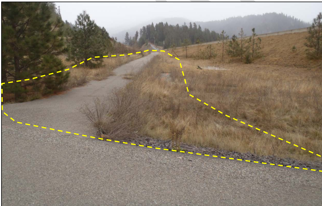
Photo 4. Looking southeast up existing 8-foot asphalt pathway. The proposed temporary on-ramp would closely follow the grade of the existing pathway from Coeur d'Alene Lake Drive to Interstate 90. Proposed temporary on-ramp footprint would be within yellow dashed line. The small wetland to the right of the on-ramp footprint would be protected during construction with erosion and sediment control measures.
