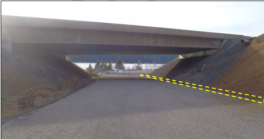
Photo 6. Looking southwest along Coeur d'Alene Lake Drive toward Coeur d'Alene Lake. Clean rocks would be placed on the west side of Coeur d'Alene Lake Drive to allow the transports to travel beneath the overpass. The placement of rock will allow existing drainage patterns to be maintained.
