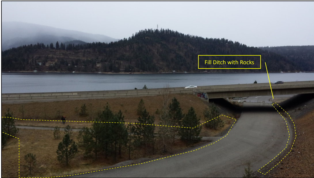
Photo 3. Looking southwest at proposed temporary on-ramp site. Proposed temporary overweight truck route would travel under I-90 and turn onto the proposed on-ramp. Clean rocks would be placed on the west side of Coeur d'Alene Lake Drive to allow the transports enough clearance to travel below the I-90 overpass. Proposed work footprints would be within yellow dashed lines.
