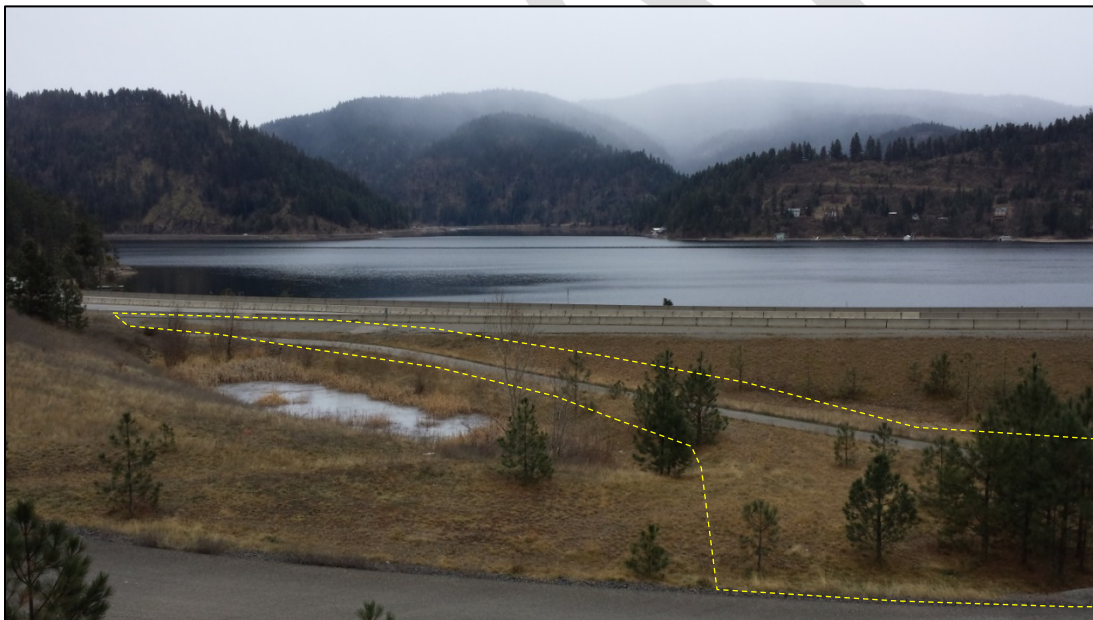
Photo 2. Looking south at the existing 8-foot wide asphalt pathway. Proposed temporary on-ramp footprint would be within yellow dashed line. Trees (mostly Ponderosa Pines) within on-ramp footprint would be felled.
